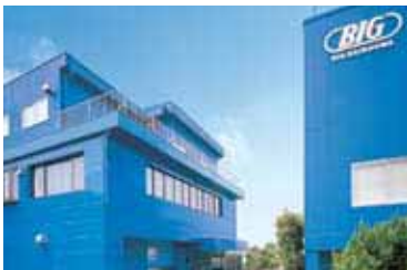
● Head Office FA Factory
